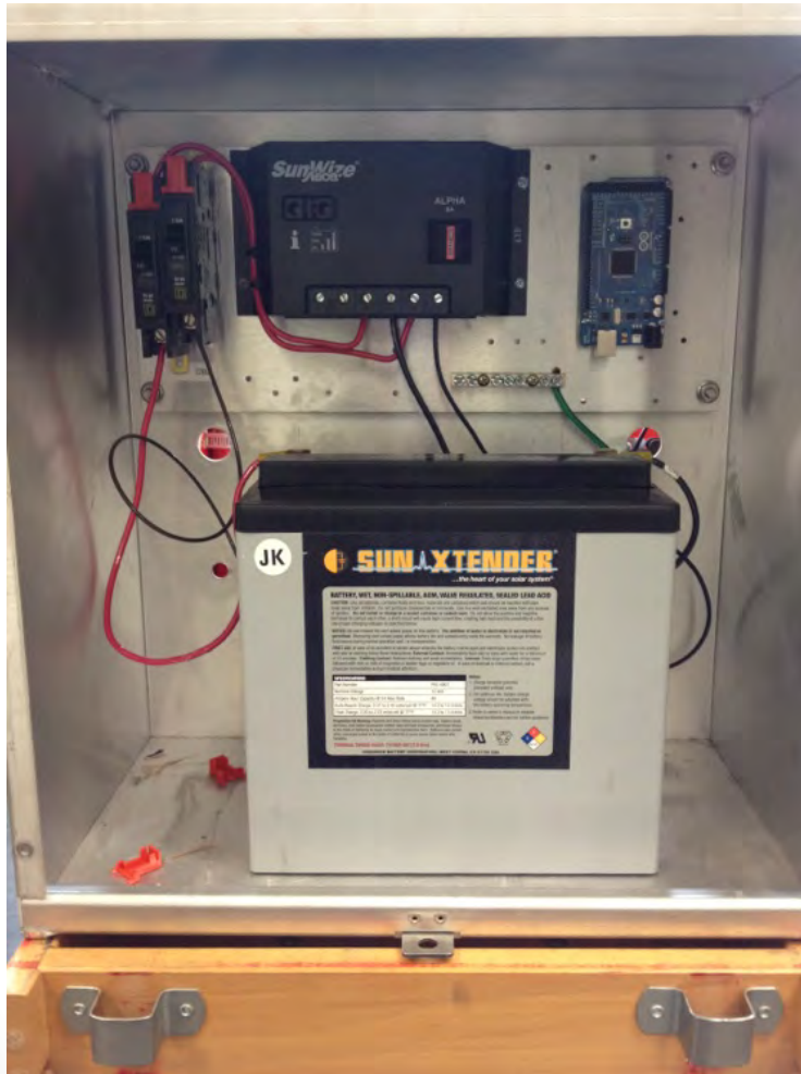
Battery, Charge Controller, Electronics
